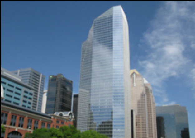
Eight Avenue Place, Calgary
