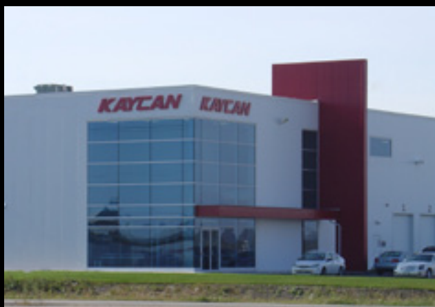
9 Davis Way, Kaycan Building, Winnipeg
